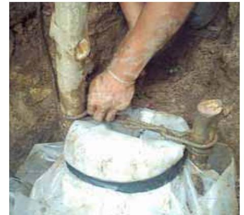
11. If necessary reposition the angle of the inlet and outlet tubes so the bottoms are well below water level and fluid can easily flow out of the digester. Tie a long piece of rope between the two vertical stakes to hold the tubes firmly in place.
